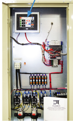
(Inside Mounted) HMI Touchscreen Control Panel for Outside Chillers
